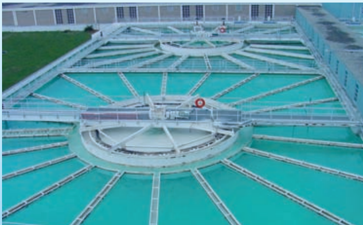
Miami Water Treatment Plant
